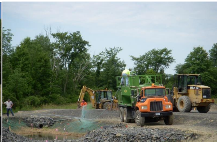
Hydroseeding Stormwater Pond Embankment
