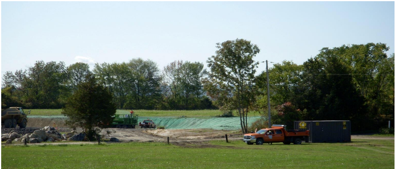
Hydroseeded Slope Stabilization
