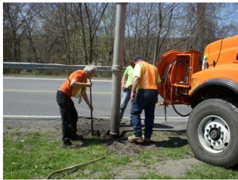
Catch Basin Cleaning
