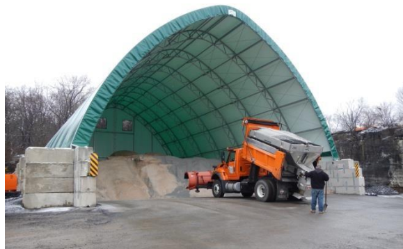
Salt Storage Shed
